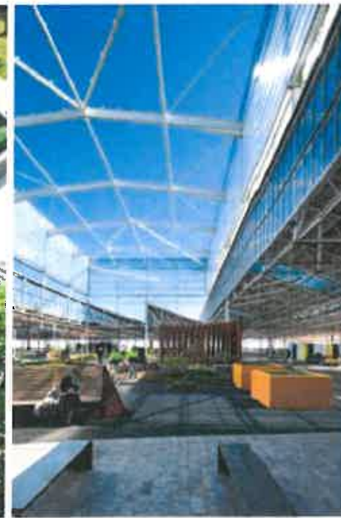
Tonsley Innovation District, Adelaide, Australia
